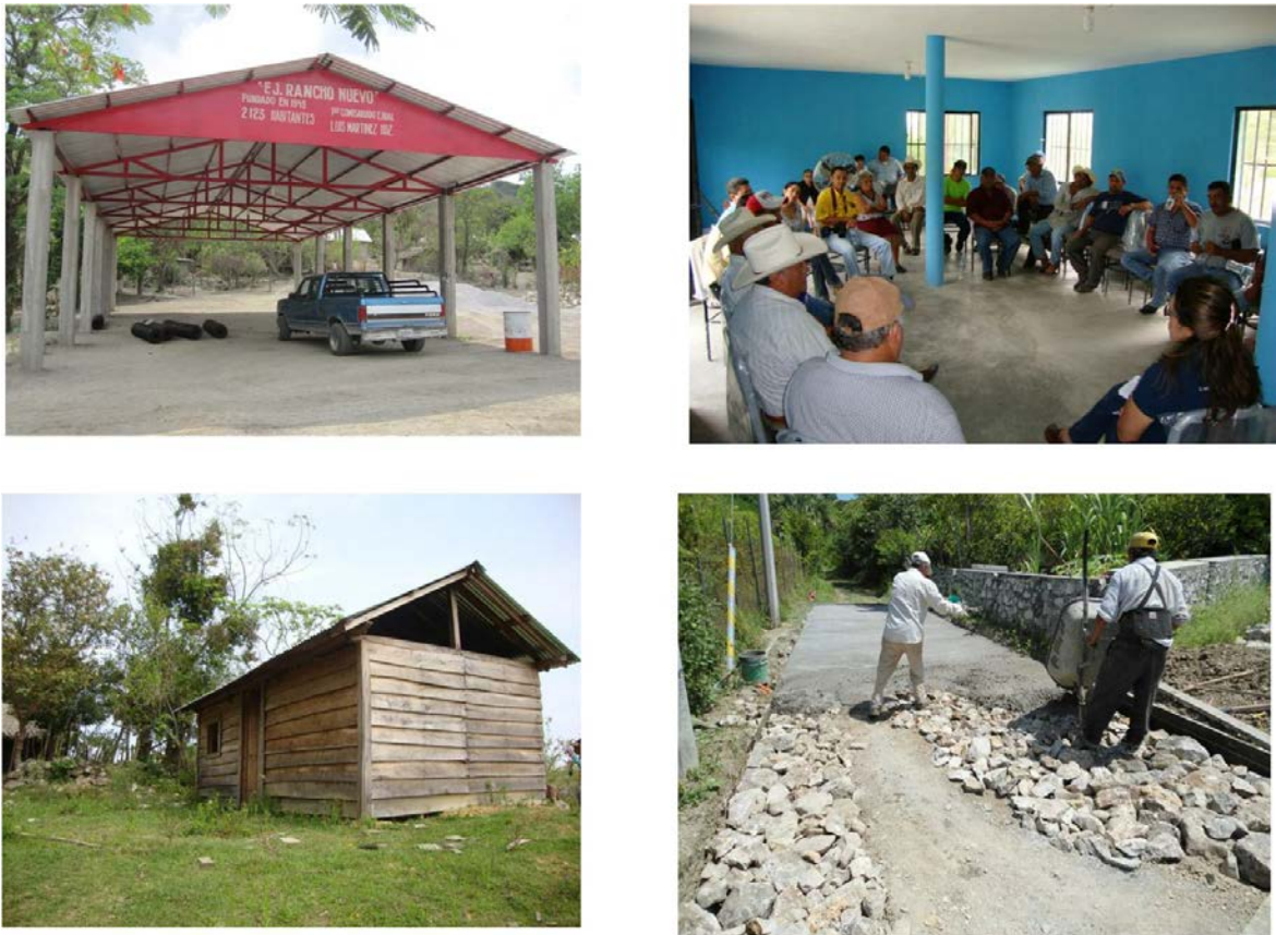
Figure 33. Infrastructure improvements using PES funding in the northern region.
