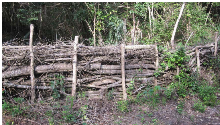
Figure 27. Fence to prevent washouts during rainy season in La Concha.
