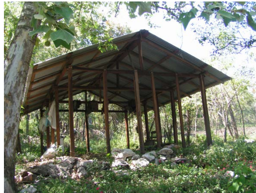
Figure 28. Roof installed in the sierra by La Concepcion with PES money.
